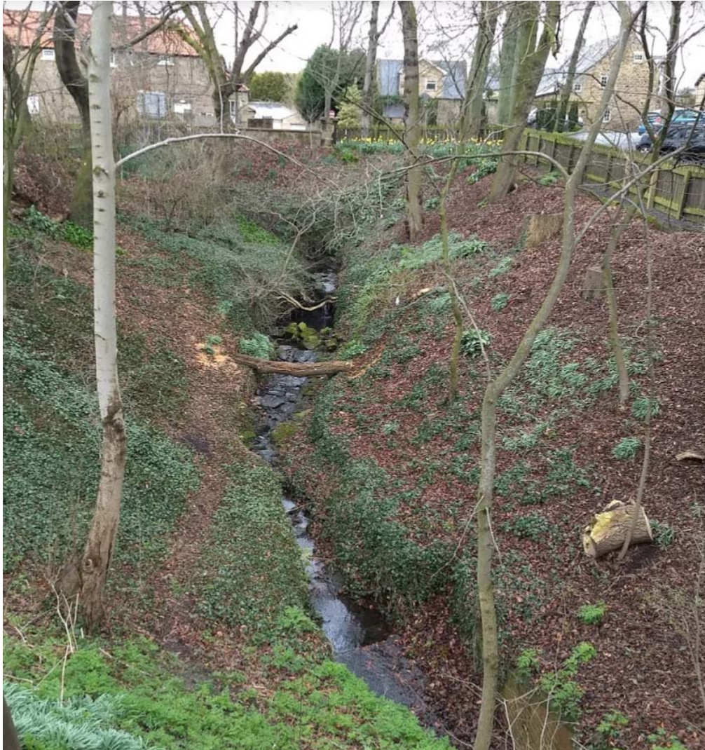
Figure 11 - View of the watercourse upstream of the culvert inlet
