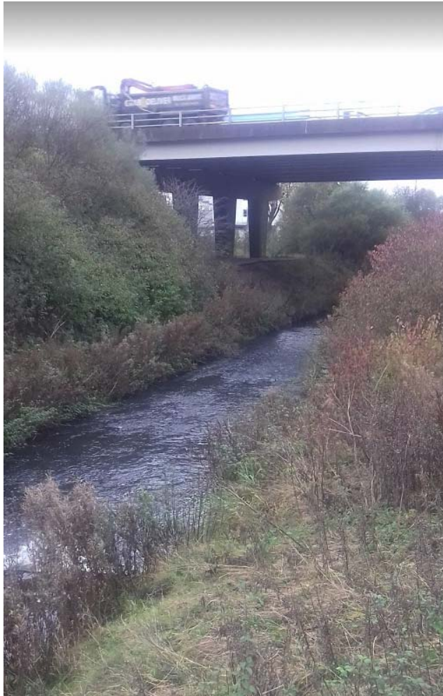
Figure 7 - View of the River Team looking downstream to the Kingsway Viaduct
